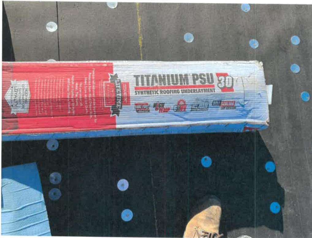
Figure 4 – Secondary Water Barrier at Sloped Section (Typical)
