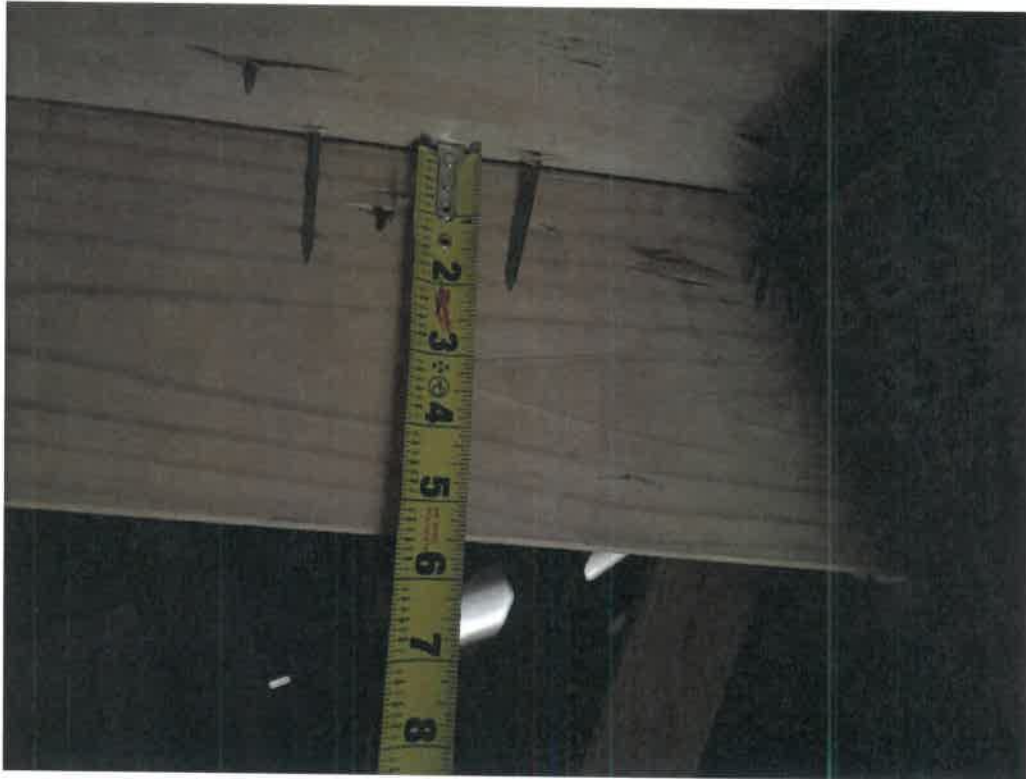
Figure 3 – Sheathing Fastener Size 8d Confirmed (Typical)
