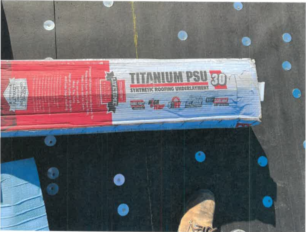
Figure 4 – Secondary Water Barrier at Sloped Section (Typical)
