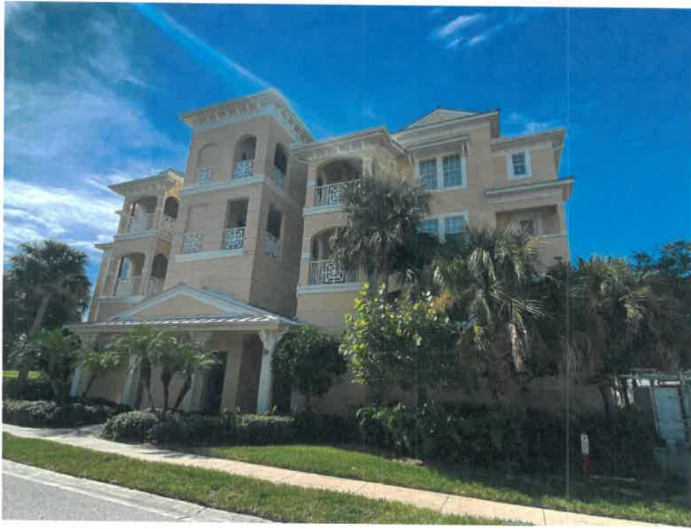
Figure 1: Typical 4-Story Roof Type (Metal) and Geometry (Hip)
