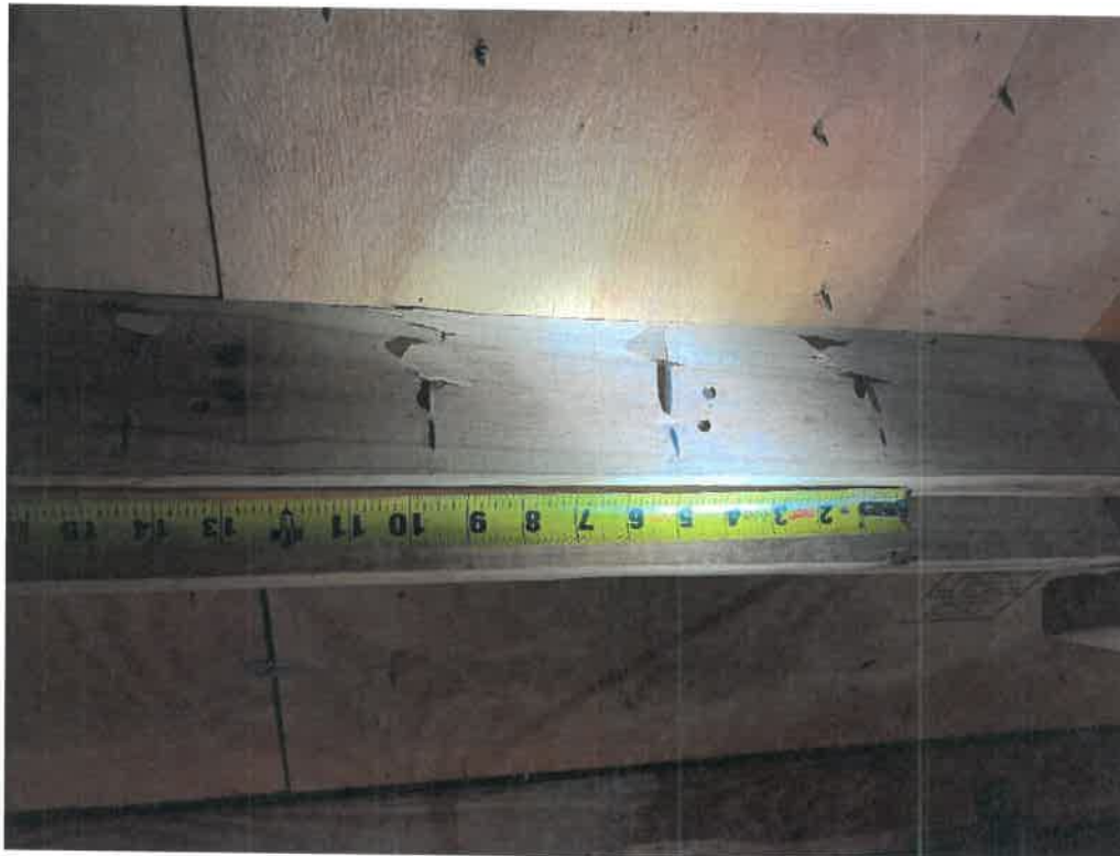
Figure 2 – Plywood Sheathing Nail Spacing (Typical)
