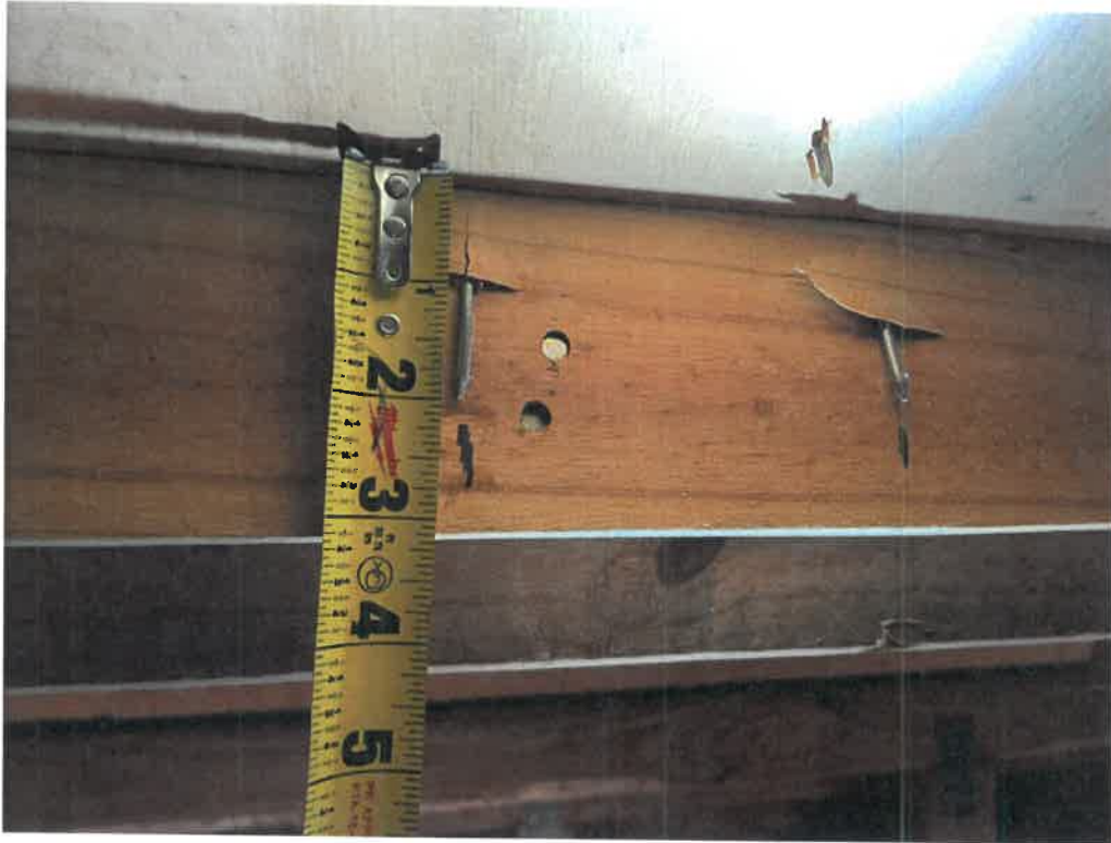
Figure 3 – Sheathing Fastener Size 8d Confirmed (Typical)
